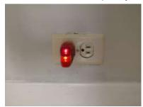
Dining Room: □ □ □ Reverse polarity is noted, Under window and at wall.
