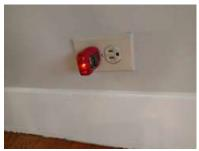
Bedroom #1: Side □ □ □ Reverse polarity is noted, Outlet between built ins.
