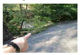
3.4 - COMMENTS: The composition shingle roofing material appeared to be in satisfactory condition relative to its age. The roof was walked on for the inspection.
