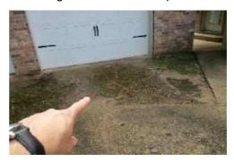
1.8 - MONITOR: The concrete driveway is functional but has some cracks that are probably due to settlement or expansion but that do not appear to warrant attention or concern at this time.
