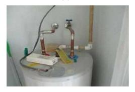
6.25 - SAFETY: There is a temperature and pressure relief (TPR) valve but no discharge line for the valve, which represents a potential scalding hazard and which can result in internal water damage should the valve ever leak. One will need to be installed and made to terminate at a visible location at the exterior of the home and within six inches of the ground.
