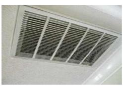
8.2 - COMMENTS: The bedroom split-system central cooling responded to normal user controls at the time of the inspection, with an average differential temperature split of approximately 18 degrees F degrees between the air entering the return and that coming out of the registers.
