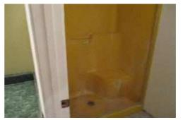
6.16 - PREVENTIVE: There is discoloration in the vinyl floor covering at the base of the hall bathroom stall shower that suggests that it may be leaking or has leaked at some time in the past. Because testing stall shower enclosures for watertightness falls outside the scope of a home inspection, you may wish to have this condition evaluated by an appropriately qualified specialist to determine if the enclosure is watertight as needed.
