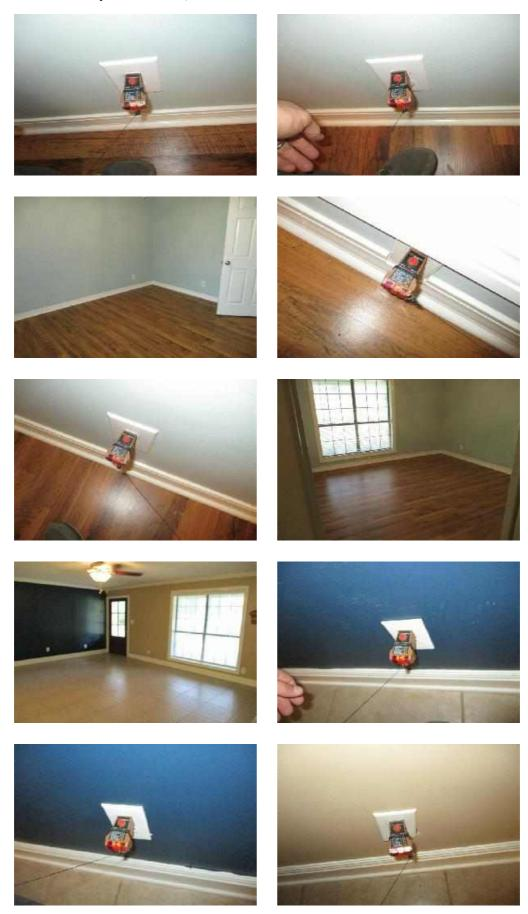
5.32 - SAFETY: There are outlets through out the home that have reversed polarity (hot and neutral wires misplaced) that will need to be evaluated by an appropriately qualified specialist and serviced for safe and proper function.
