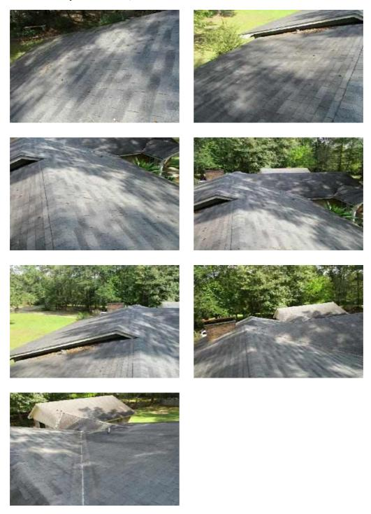
3.4 - MAINTENANCE: There are leaves or debris in some of the valleys that need to be cleared off to help prevent premature deterioration of the coverings and to facilitate drainage.
