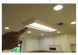
5.27 - COMMENTS: A light fixture in the back bathroom did not respond, and should be fitted with a new bulb and retested for proper function.
