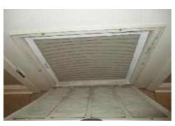
7.6 - COMMENTS: At the time of the inspection, the air filter was clean or relatively clean and did not need replacement. However, it is important to replace or clean the filter (depending on type) every two or three months. If filters are not changed (or cleaned) regularly, the ducts can become contaminated, and can be expensive to clean or replace.
